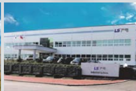
Dalian factory (China) MV/LV switchgear, MV contactor
