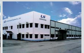
Hanoi factory (Vietnam) MV/LV switchgear, Mold TR
